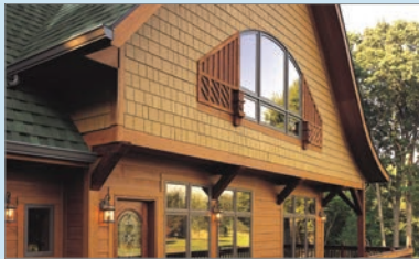
Fiber Cement Siding
